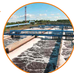
Sewage treatment plant
